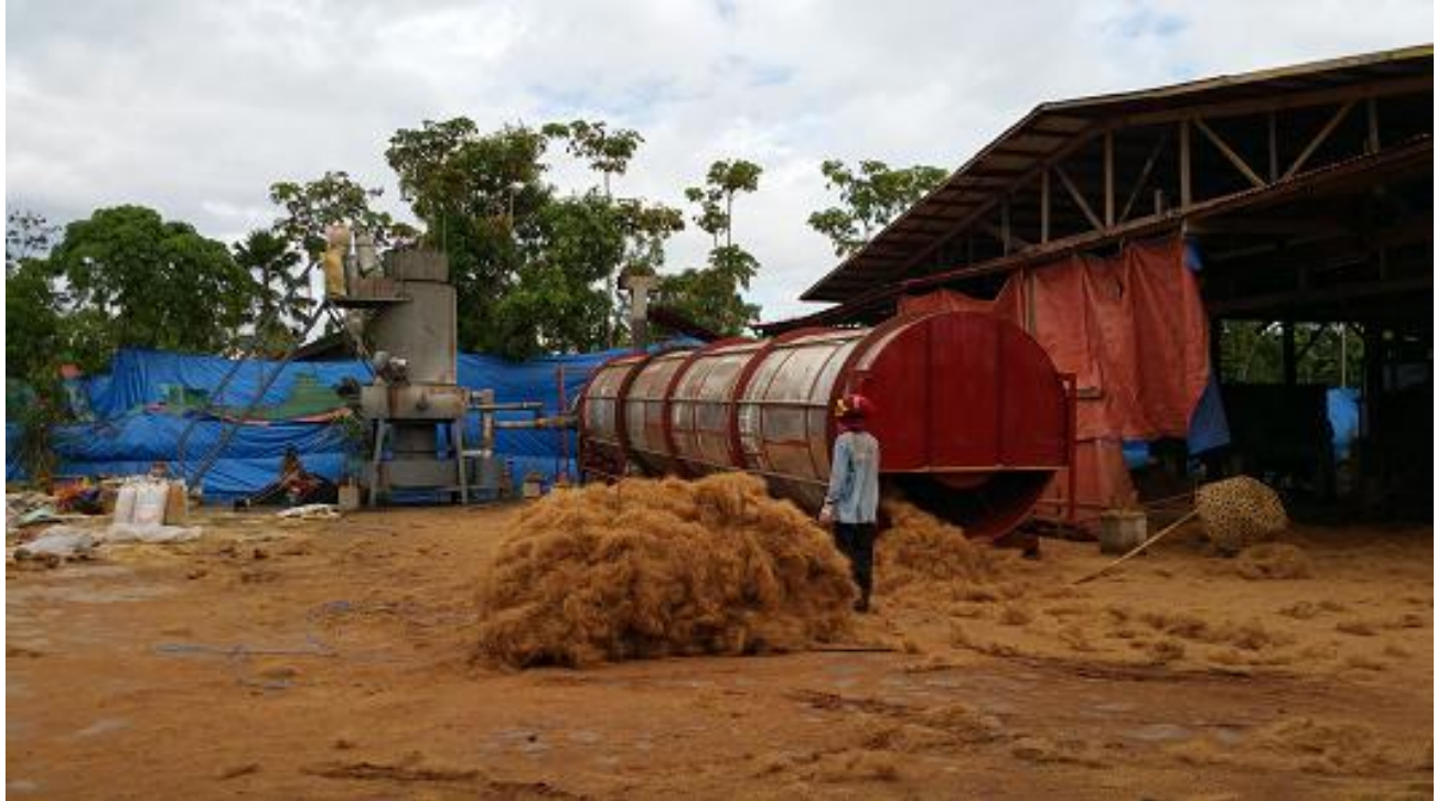
Figure 2. The Rotary Drum Dryer for Drying Coco Fiber
